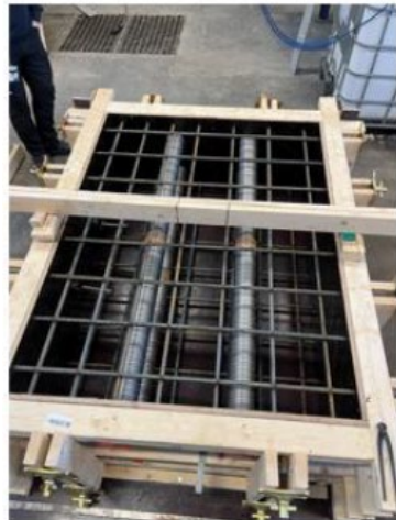
Duct placement in formwork
